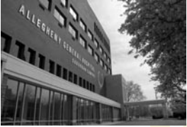
Allegheny General Hospital – Suburban Campus
